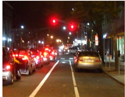
The 6" bike lane lines on Hampshire Street in Cambridge are clearly more visible than the 4" stripes adjacent to the parking lane.
